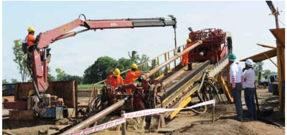
A crossing being completed with horizontal directional drilling.
