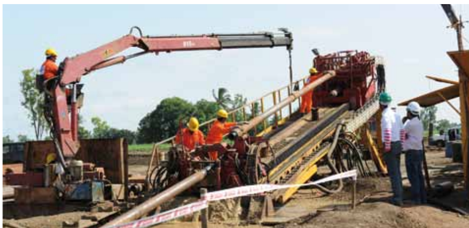
A crossing being completed with horizontal directional drilling.
