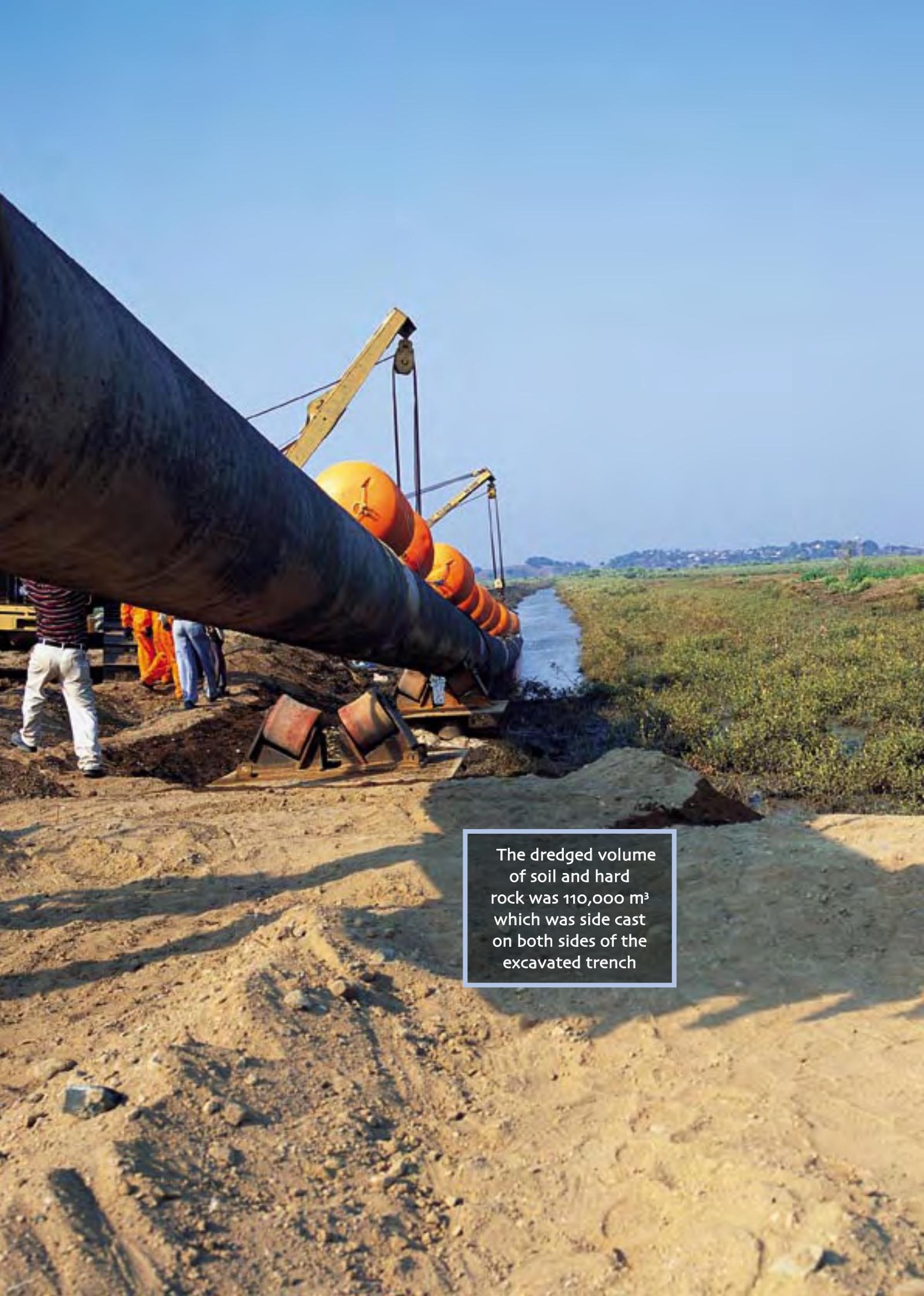
The dredged volume of soil and hard rock was 110,000 m<sup>3</sup> which was side cast on both sides of the excavated trench
