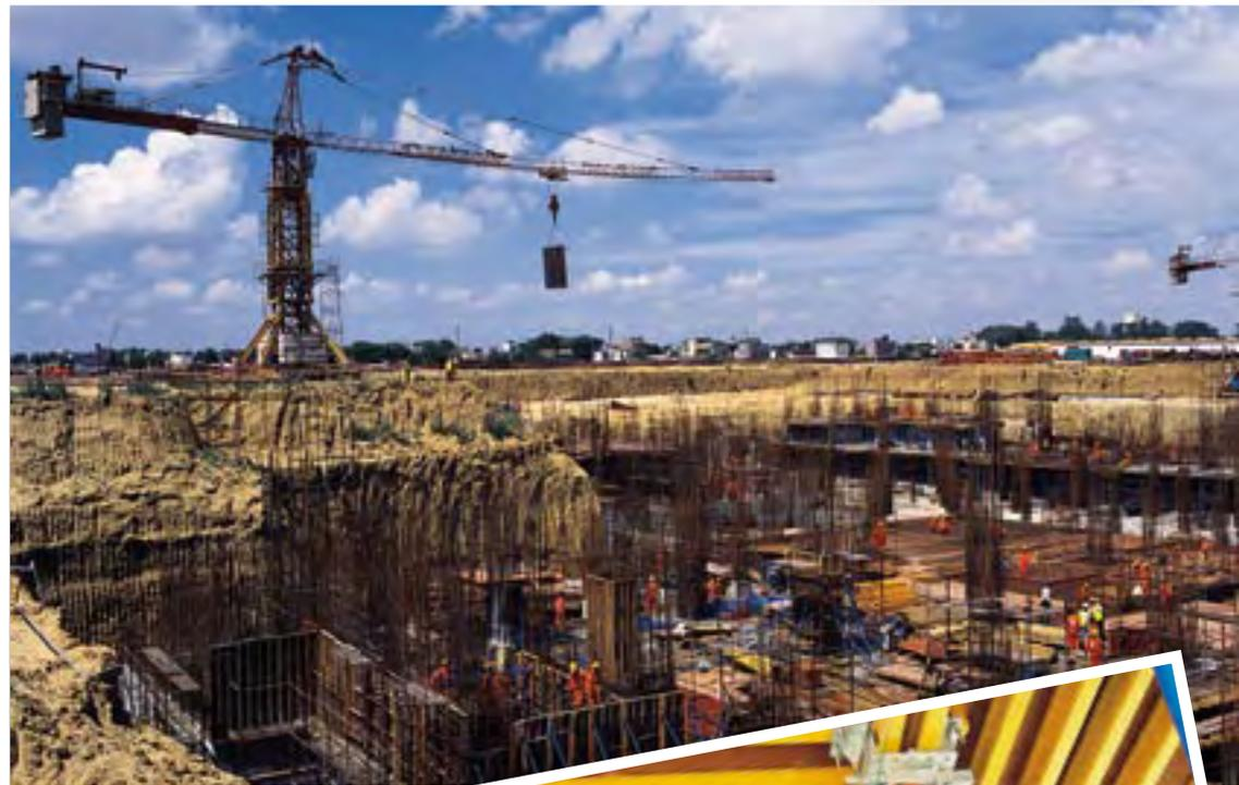
upper ground floor. The basement footprint of 18,000 m<sup>2</sup> sits on a 2 m thick raft foundation for tower blocks whereas other blocks have thickness varying from 0.3 to 0.9 m.
