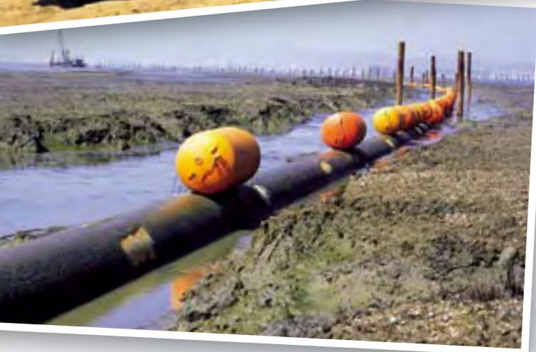
30" dia tee-off (on the Uran-Trombay pipeline) from Sheva south to JNPT Terminal, including all related onshore facilities. From upstream the oil is transported from Mumbai High and Heera and Neelam fields to Uran through submarine trunklines.
